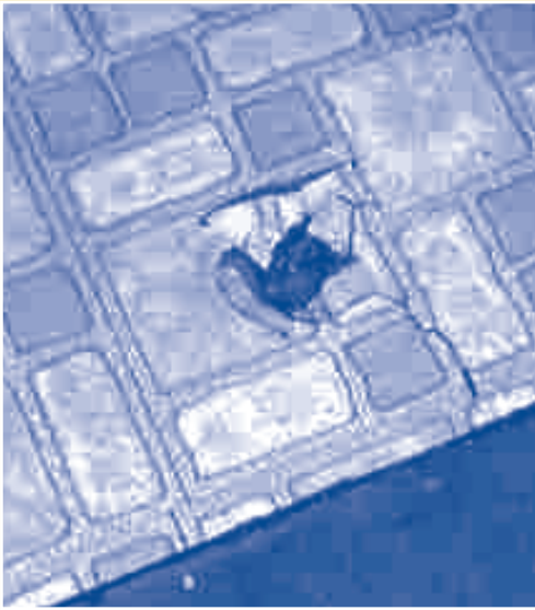
Going through the kitchen floor. Survey 2004
